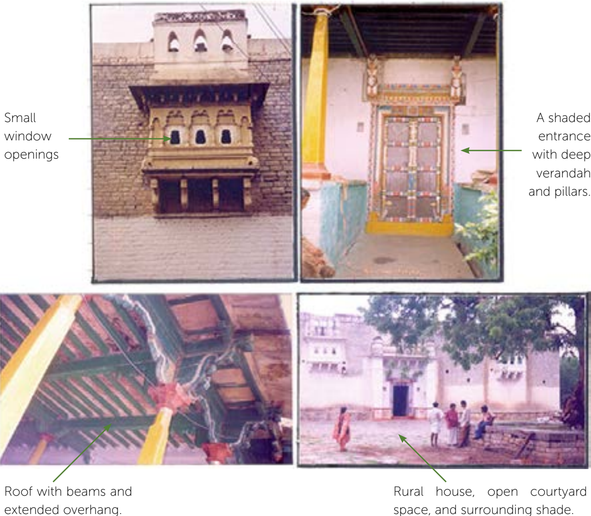
FIGURE 7 Cooling features of traditional rural houses in Kalaburagi, Karnataka
