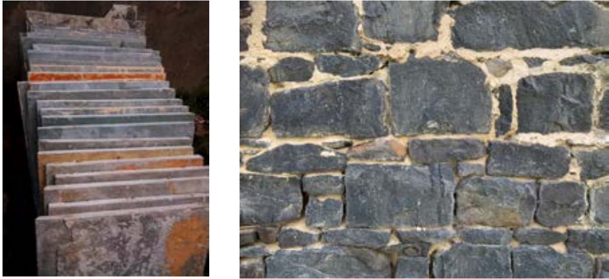
FIGURE 8 Basalt and Shahabad stone masonry bonded with lime mortar
