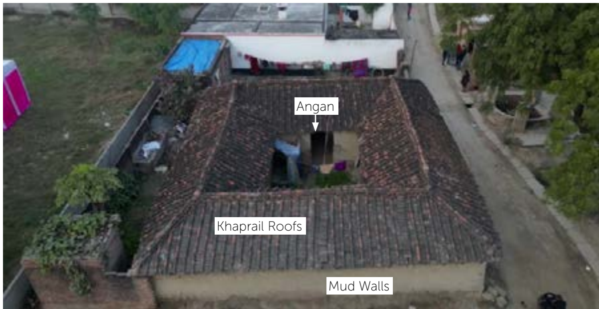
FIGURE 20 Typical rural house with khaprail roofs, mud walls and open courtyard called “Angan”
