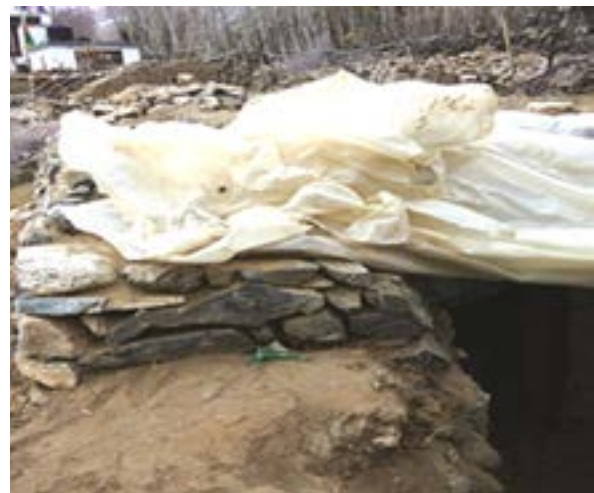
FIGURE 61 Traditional cold cellars, known as Tsothbang, used for winter storage of vegetables and grains in the Ladakh region 107
