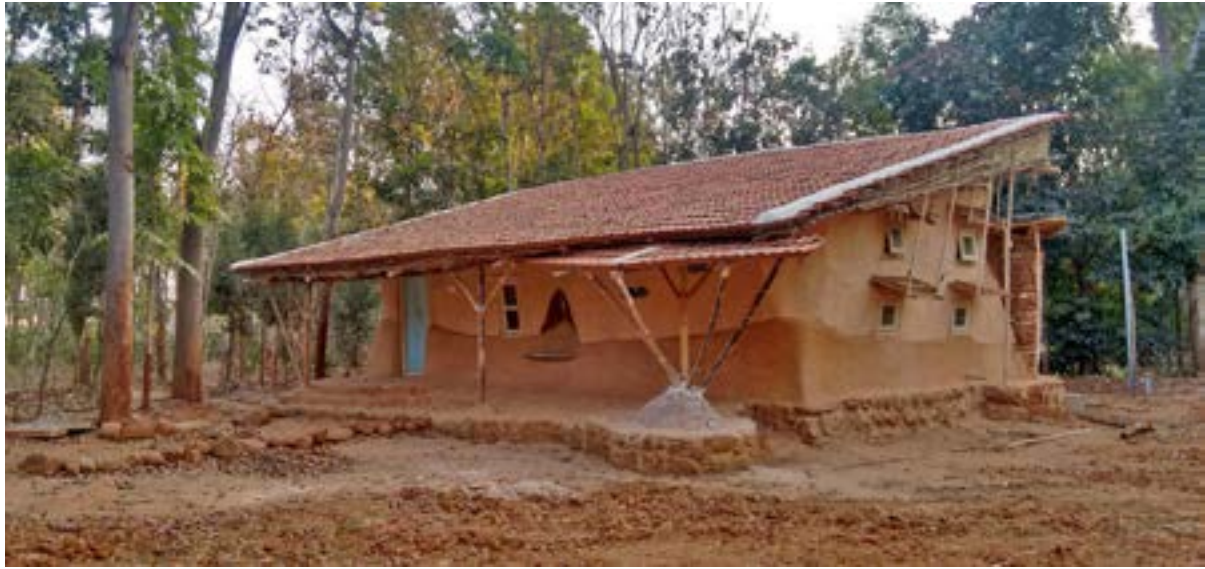
FIGURE 14 Mud Wattle daub Construction in Warm and Wet Regions of India
