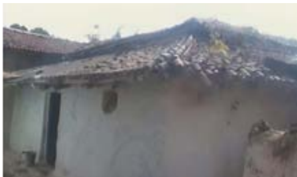
FIGURE 21 Typical huts in Jharkhand with Mud wall and khaprail roof 29
