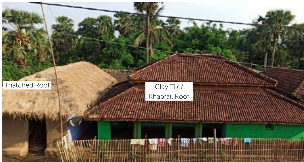
FIGURE 19 Clay tile and thatch roofing in a typical rural houses in Bihar
