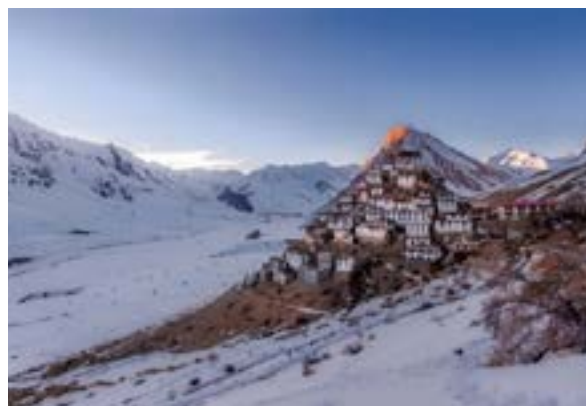
FIGURE 33 Spiti Valley settlements located on elevated platforms to reduce ground moisture and mitigate the associated frost pockets 64
