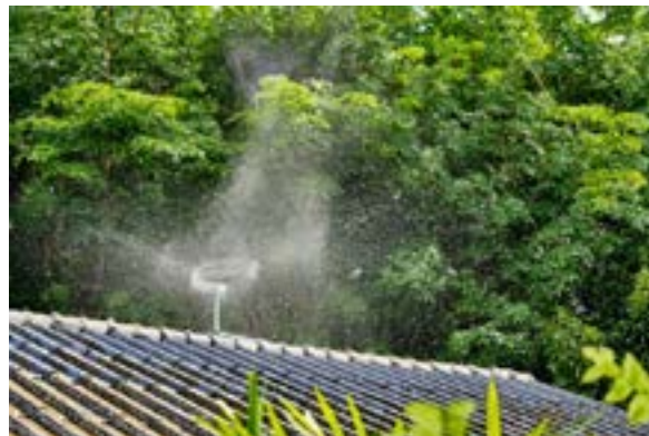
FIGURE 43 Rooftop sprinklers in rural India reducing daytime roof temperatures through evaporative cooling 79
