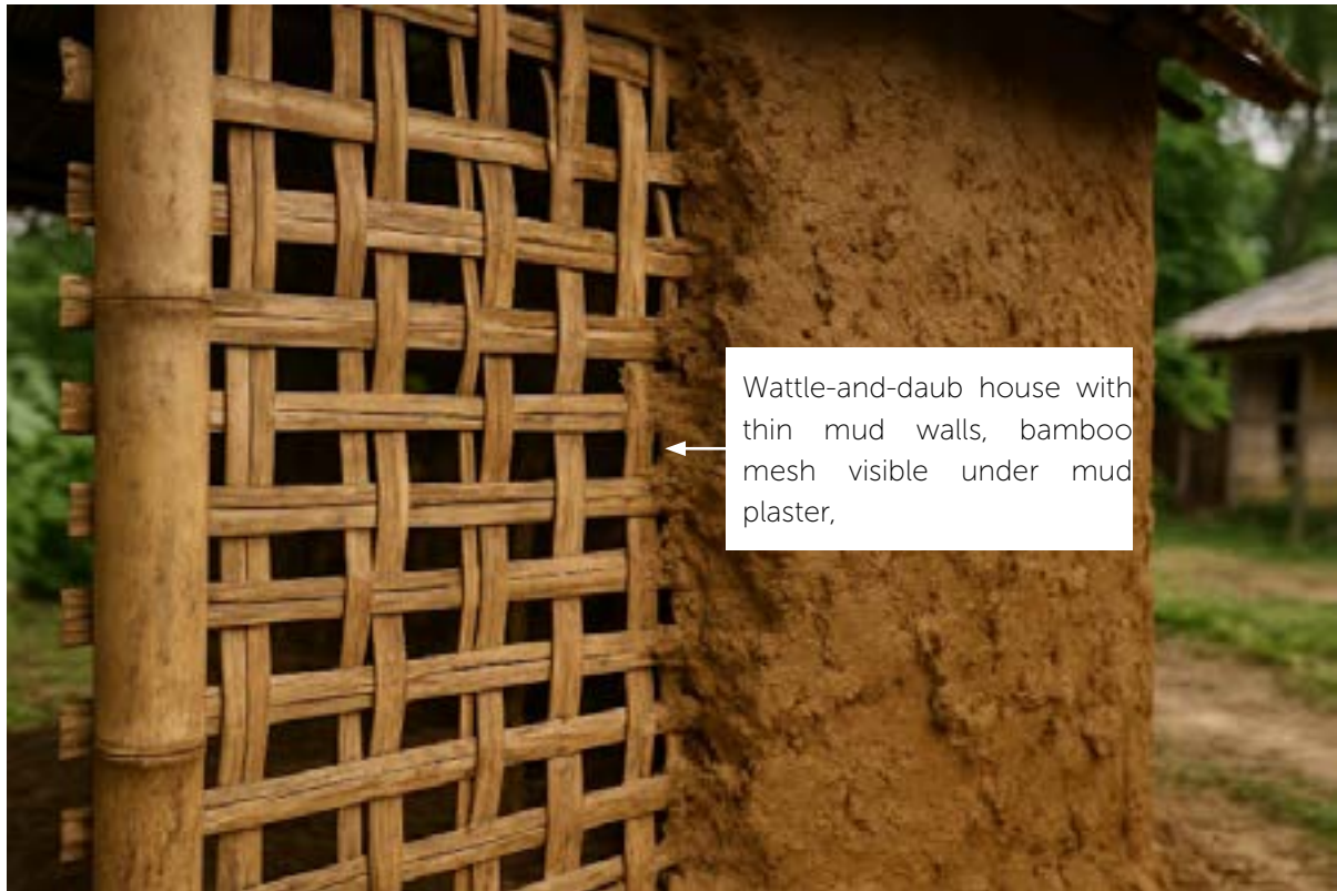
FIGURE 13 Traditional wattle-and-daub wall showing woven bamboo mesh and mud plaster.
