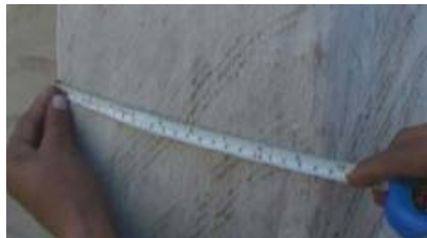
FIGURE 22 450 mm thick mud wall 29
