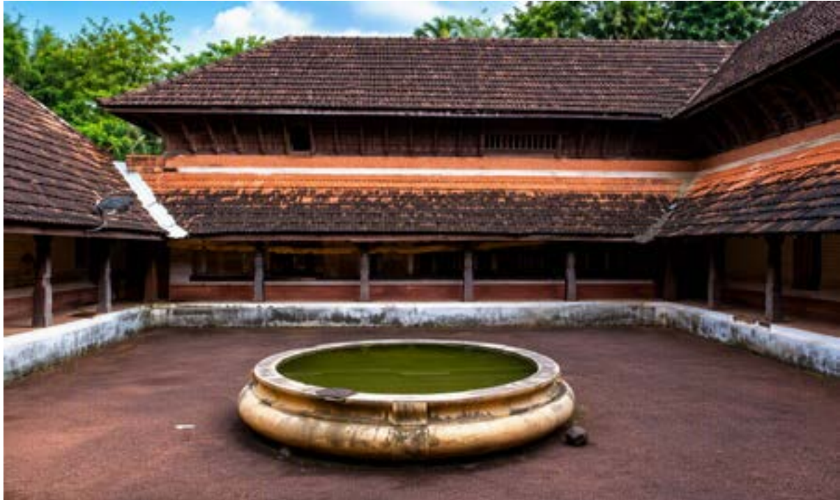
FIGURE 11 Traditional residence in Kerala with laterite stone, timber and Mangalore clay tiles
