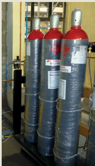
Figure 10.3 Storage of Refrigerant Cylinders
