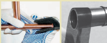
Figure 5.7 Cleaning (L) and Polishing (R)
