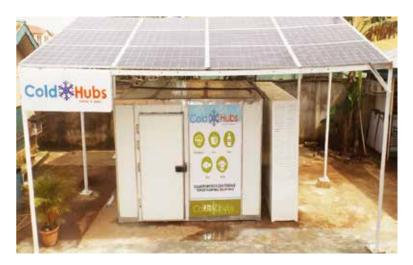
Figure 14: ColdHubs storage for fruit and vegetables based on photo voltaic and battery backup for cooling at night
