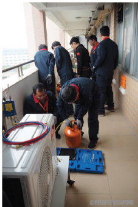
Figure 19: Refrigerant charging training
