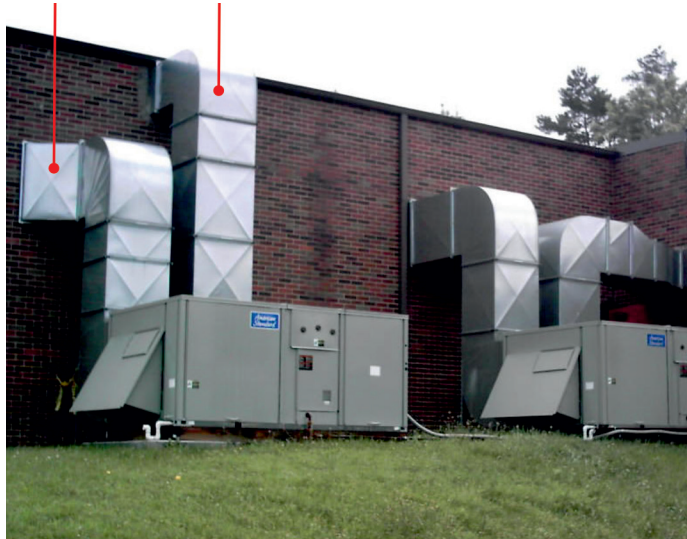
Figure 30. A 10-ton packaged air-conditioning unit
