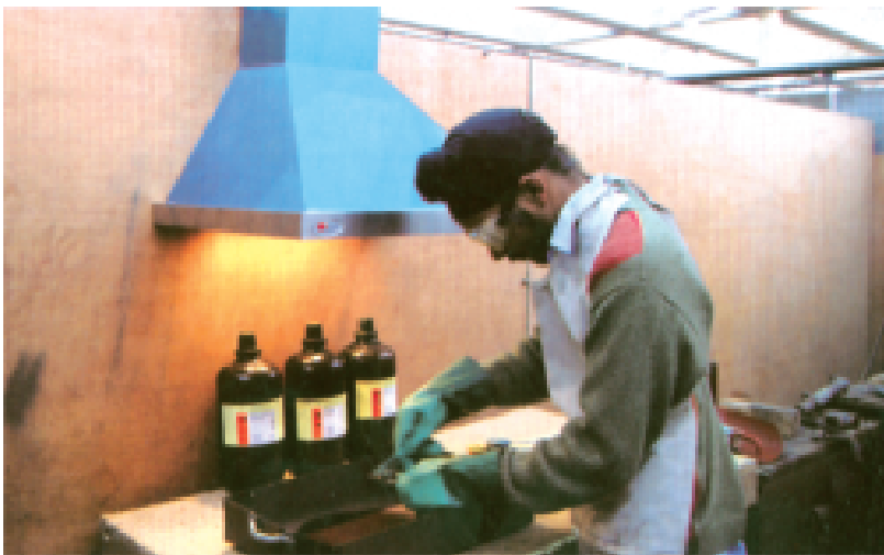
Picture 14: Local Exhaust Ventilation
