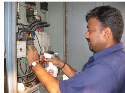
Figure 6: Cleaning of electrical contact by spraying followed by wiping method
