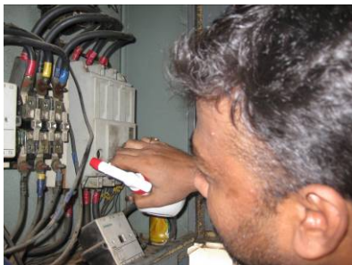
Figure 5: Cleaning of electrical contact by spraying method
