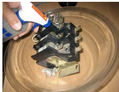
Figure 4: Cleaning of electrical contact by spraying method
