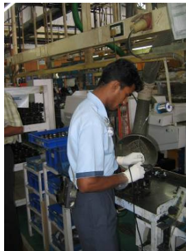
Figure 14: Stationary LEV with flexible duct
