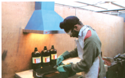
Picture 4: Local exhaust ventilation
