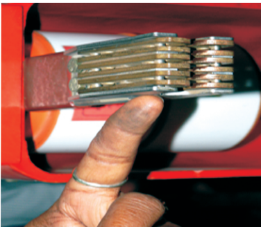
Picture 8: Cleaning of contacts
