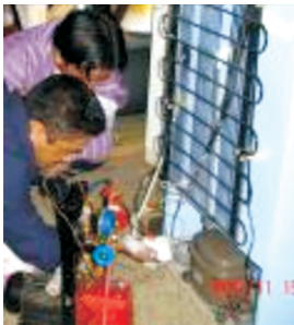
Picture 5: Refrigerator system repair
